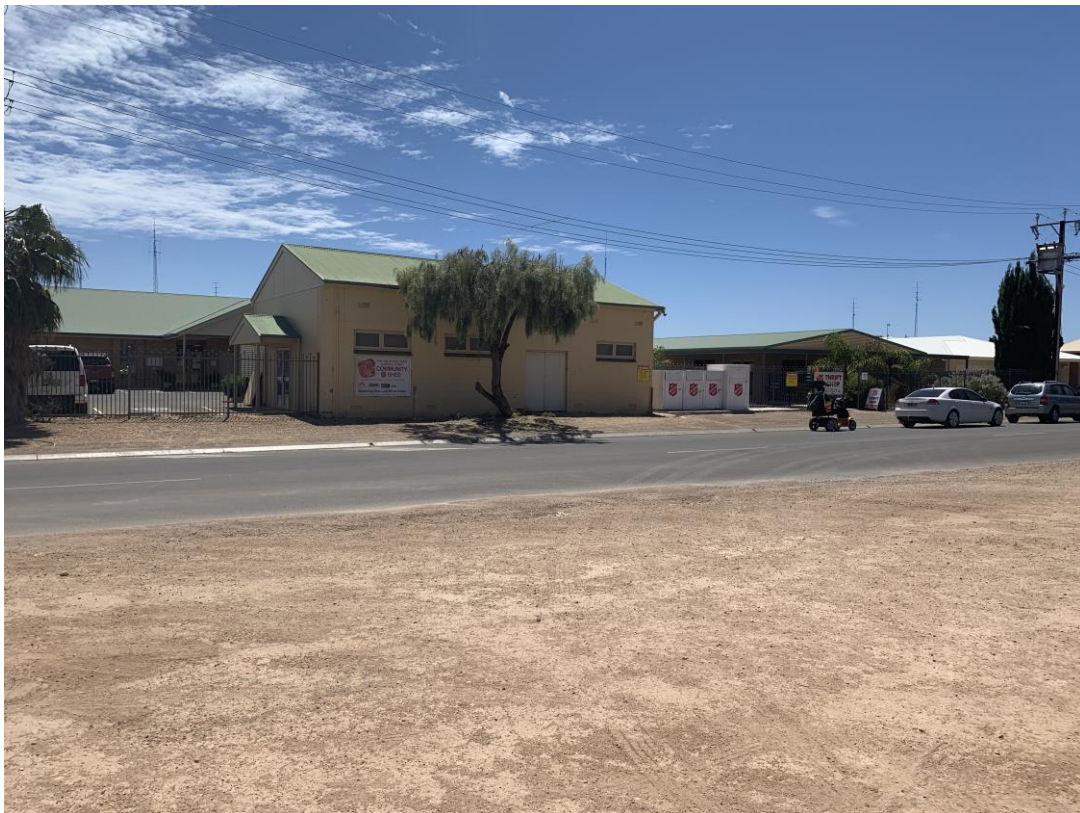
Figure 4 – Subject site from Drain Road, Kadina
