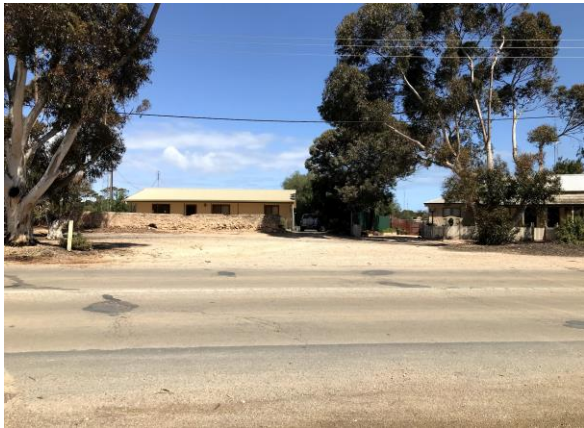
Photo 3 – Opposite subject land – looking south
