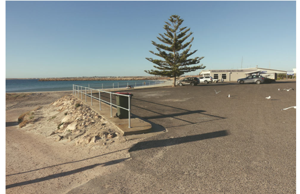
Existing site condition
