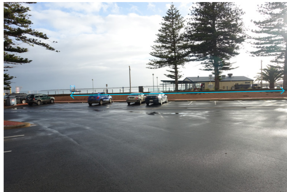
Adjacent gradient, lack of surface and connection creates physical barrier.
