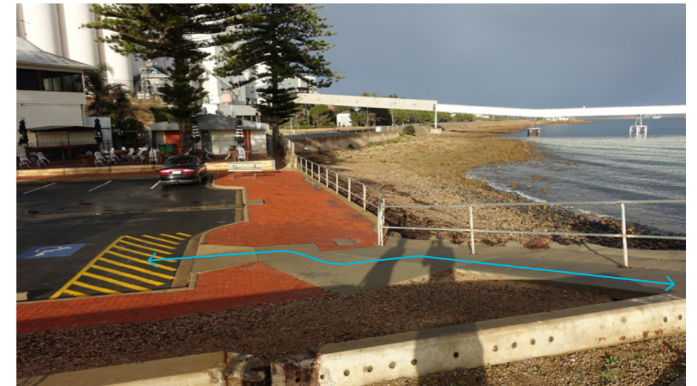
Physical barriers from accessible car parking limits access and requires users to find alternative route. Car parking set out non-compliant to current standards
