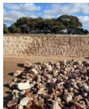
Front Wall – Part of the wall has been removed with the rebuild the lighter colour stone.
