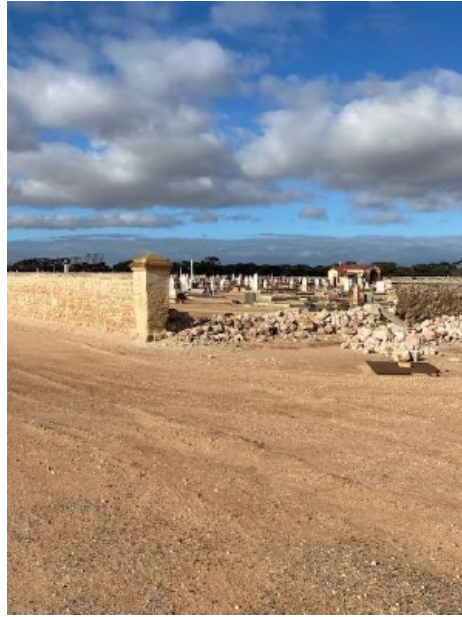
Back Wall Northwest corner Recently collapsed, will require rebuilding as an anchor for the corner pier.
