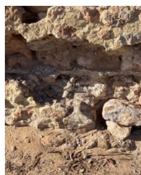
Front Wall – Portion of the front wall that is required to be rebuilt. There is around 15m of front wall still to be rebuilt before getting repointed.
