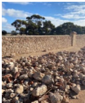
Front Wall – Part of the wall has been removed with the rebuild the lighter colour stone.
