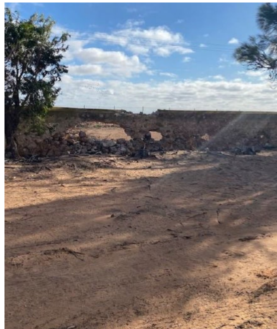
Back Wall Northwest corner Recently collapsed, will require rebuilding as an anchor for the corner pier.
