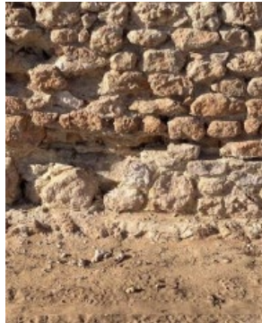
Front Wall – Portion of the front wall that is required to be rebuilt. There is around 15m of front wall still to be rebuilt before getting repointed.
