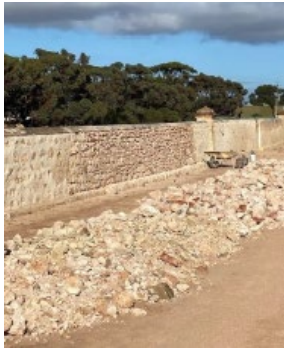
Front Wall – Part of the wall has been removed with the rebuild the lighter colour stone.
