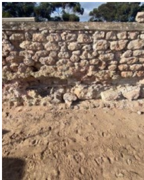
Front Wall – Portion of the front wall that is required to be rebuilt. There is around 15m of front wall still to be rebuilt before getting repointed.
