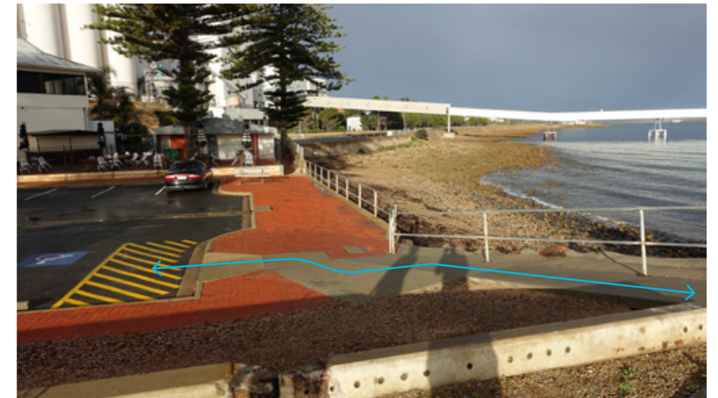
Physical barriers from accessible car parking limits access and requires users to find alternative route. Car parking set out non-compliant to current standards
