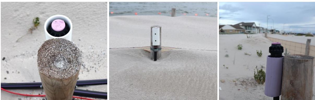
Figure 32: An irrigated sprinkler system can be used to wet sand and stabilise dunes during strong wind conditions; they also promote rapid vegetation growth.
