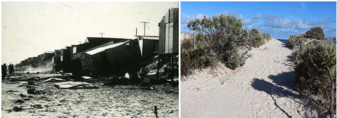
Figure 5: Storm damage at North Glenelg (left); an intact dune system at Tennyson Beach that absorbs storm damage, enhances amenity and reduces risk of storm damage (right).
