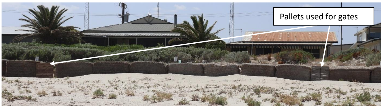
Figure 29: Pallets are a readily accessible and affordable option for temporary gates that also reduce wind erosion of the dune
