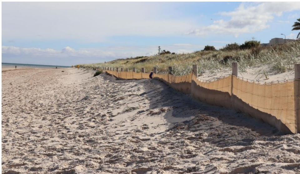
Figure 24: A staged installation of drift fencing can be used to build a dune.
