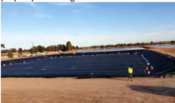
High-density polyethylene lining lagoon 1A
