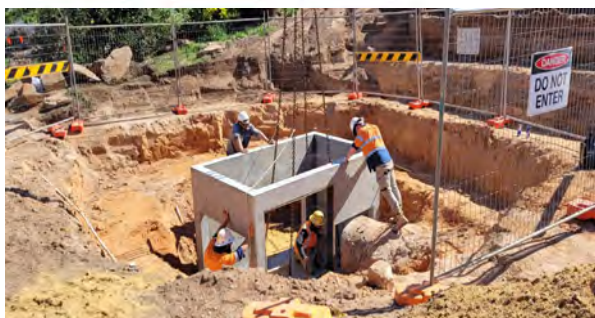
Installation of pits for Bay Road stormwater, Moonta Bay.
