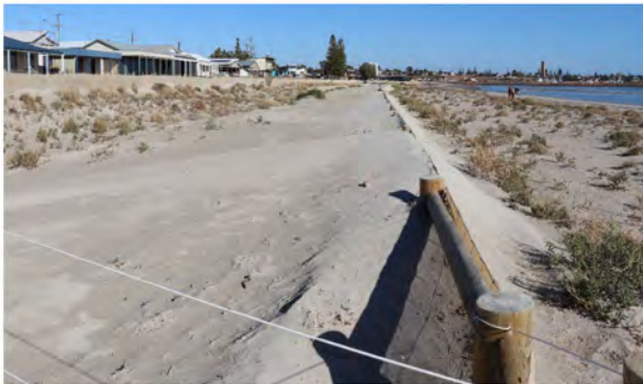
Sand dunes forming over the new fences to stop the build-up of sands over beachfront properties on North Beach
