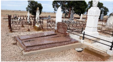
Reactive soils/inadequate foundations
