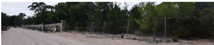
Eastern side fence extension in cyclone wire
